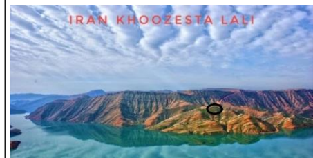
Figure (7): Pictures of the project location and its view on the GOTVAND Dam Lake
