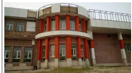
Figure (6): Pictures of the construction site
