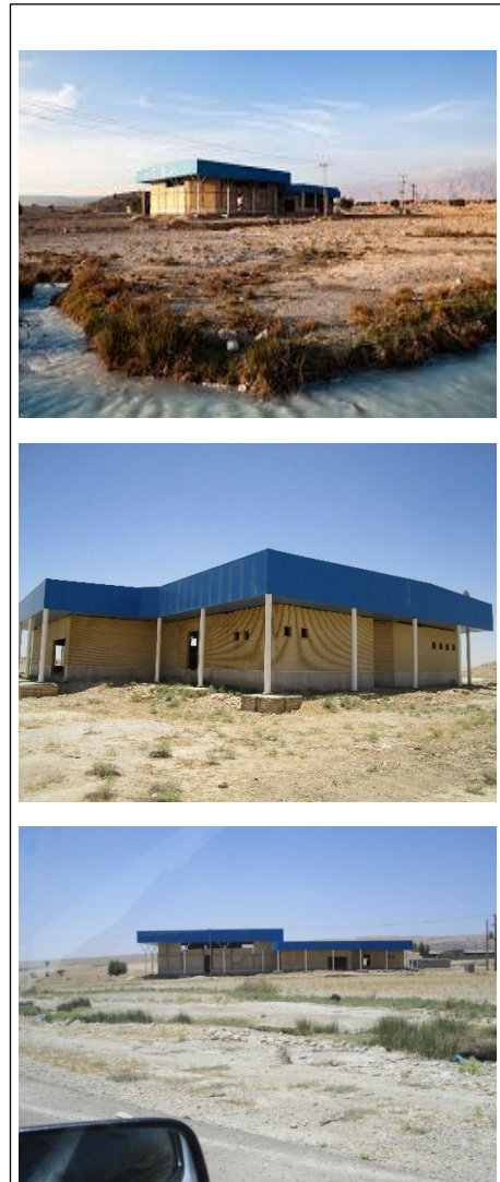
Figure (6): Pictures of the construction site
